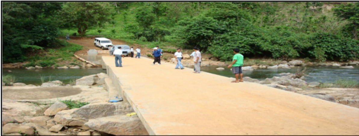
Causeway Bridge constructed through convergence in West Garo Hills, Meghalaya
