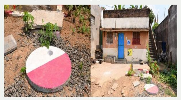
**Individual household soak pits** are simple to construct with locally available materials. Under this system greywater can be treated at source, preventing the flow of greywater onto the village paths, open land or stagnating in low lying areas. In Pappankuzhi village, 93 households could not be connected to the drainage channel and hence were provided with individual household soak pits to manage grey water.
