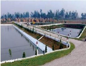
A waste stabilization pond (WSP) is a series of shallow man-made basins that facilitate digestion of organics in the greywater through natural processes within the stipulated retention time. A WSP comprises of anaerobic, facultative, and maturation ponds. (Manual on Greywater Management – DDWS)
