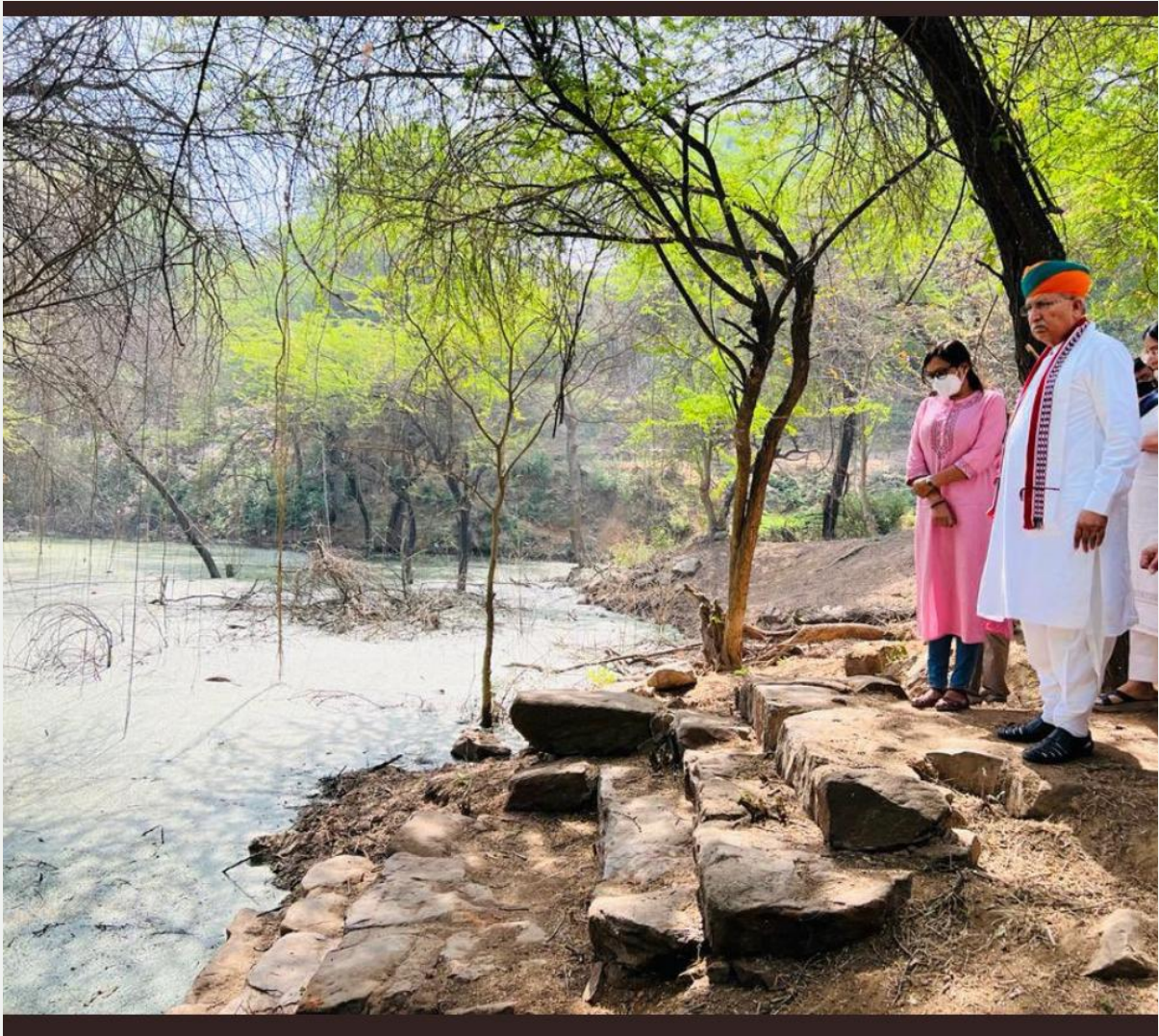
Shri Meghwal was surprised to see the dilapidated condition of the millennium old Anang Tal which signifies the beginning of Delhi. He instructed to finish the work of cleaning of Anang Tal
